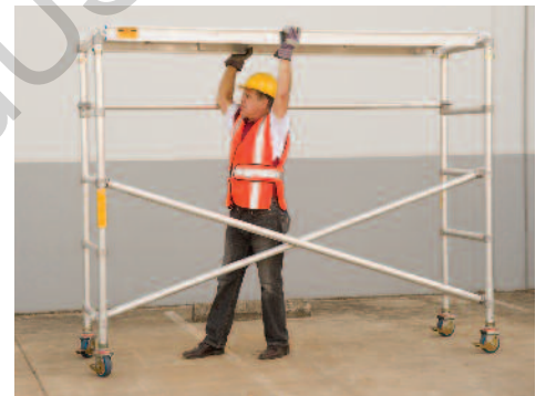
3. Install platform at desired height.
