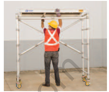
4. Install platform at desired height.
