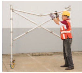
3. Lock hinging braces (see "Locking hinges" on page 3).
