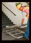
It requires no tools and can be erected to multiple heights in five simple steps using the base section, the platform and standard aluminum components.
