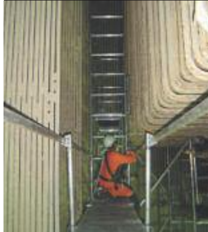
Above Left: Superheater Access Platform. Provides access for operators between superheater platforms.
